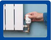
Don't turn thermostatic radiator valves off, always keep them on a minimum frost setting.
